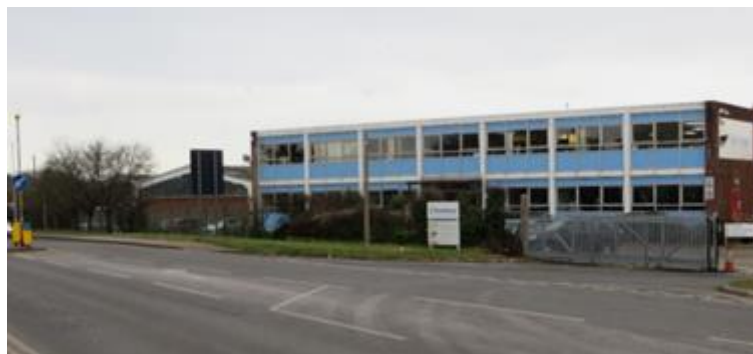
View of front of site (Source: Design and Access Statement)
