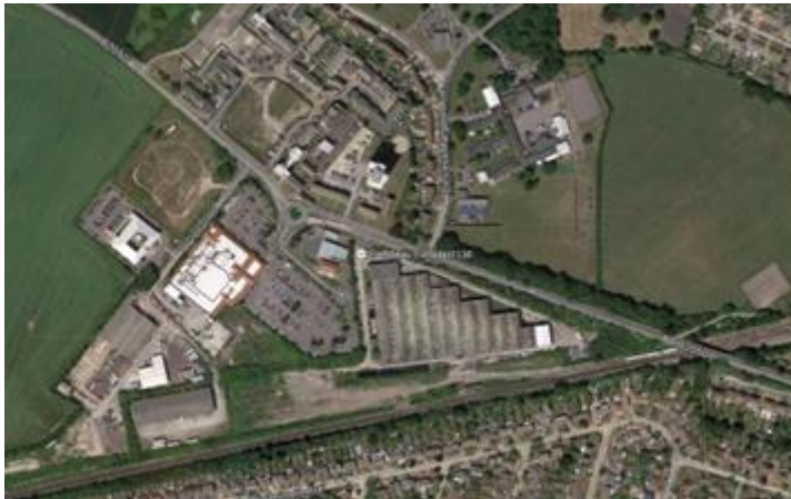
Aerial view of site (Source: Design and Access Statement)
